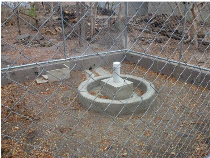
Well is capped until the pump can be installed.
